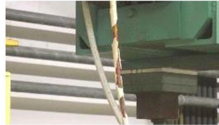
Cabling status inspection
