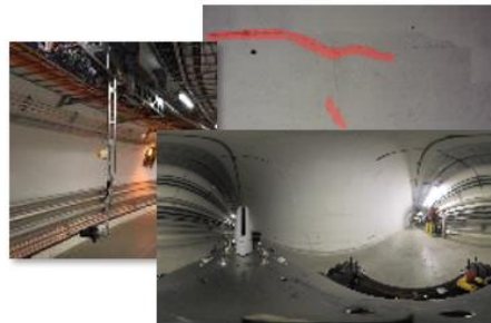
Tunnel structure monitoring
