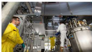
Upgrading the TS1 Target Service Area
