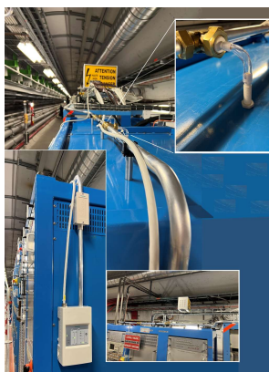
Fig. 4 - Typical Pipe and ASD Installation
