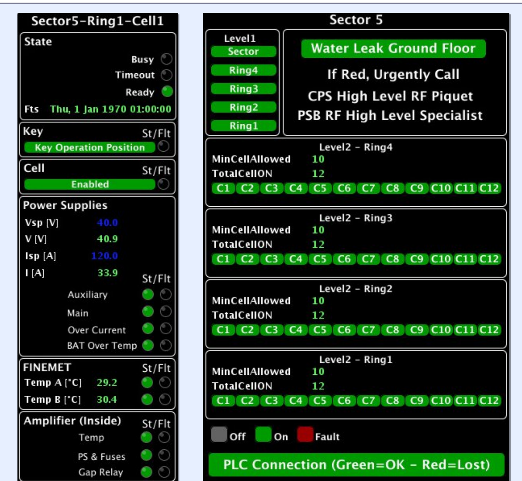
Monitoring panel for the ring 1 in sector 5 (left) and the general view panel for sector 5 (right)
