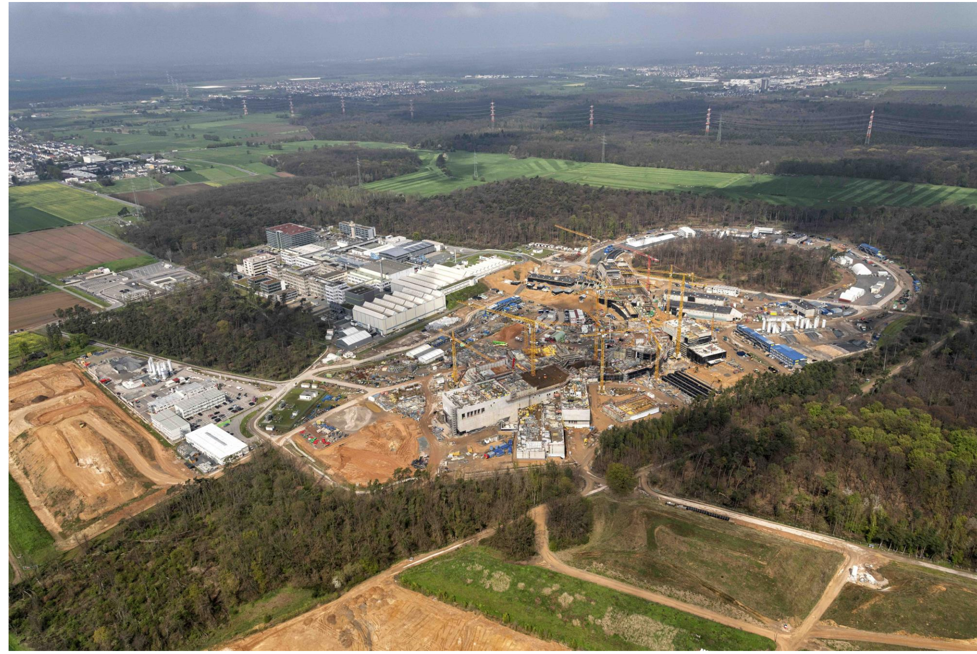
Figure 1: Aerial view of the FAIR construction site in April 2023 (Photo: D.Fehrenz/GSI/FAIR)
