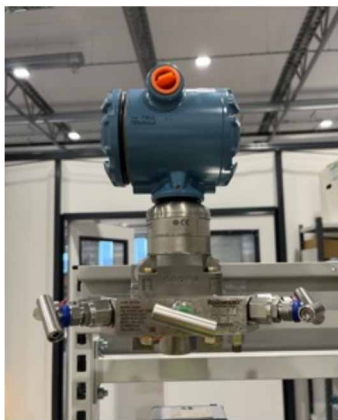
Figure 3: Mass flow measurement instrumentation, the manifold is He tight.
