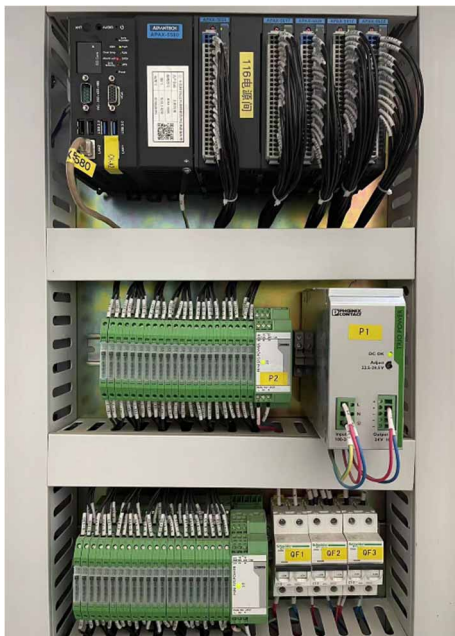
Figure 3: The power supply control system hardware.
