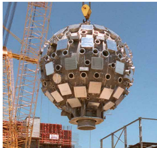
Figure 3: Target chamber at NIF before installation, the 192 beams enter in groups of 48 quads (seen as the capped squares on the chamber’s surface above).
